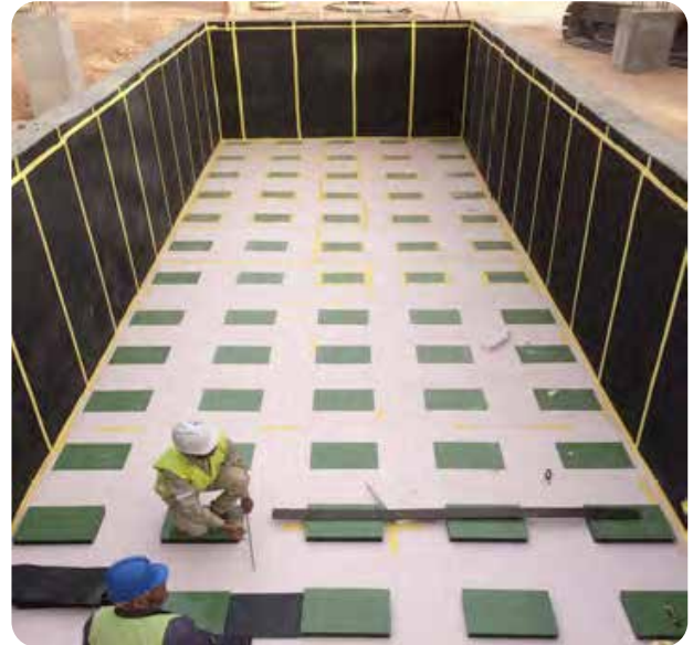
Fig 7.2 Example IFD Pit Using ISOMAT
