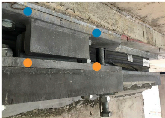
Figure 9: Vibration measurements taken across the (Farrat) bearing assembly that incorporates elastomeric LNR Bearings, fail safes, vertical continuity ties and lateral restraints. A reduction of over 20 dB is shown across the key 40 – 100 Hz range.
