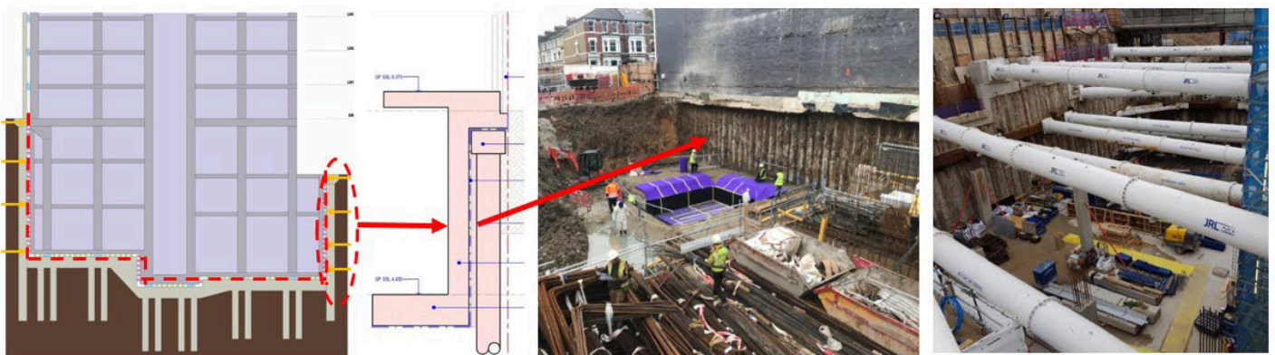
Left to right: Figure 1a: Indicative 'full area' building isolation system for a deep basement, Figure 1b: Acoustically separated double wall (retaining and inner liner) design, Figure 1c: Construction of design shown in Figure 1b, Figure 1d: Example of a deep basement construction.
