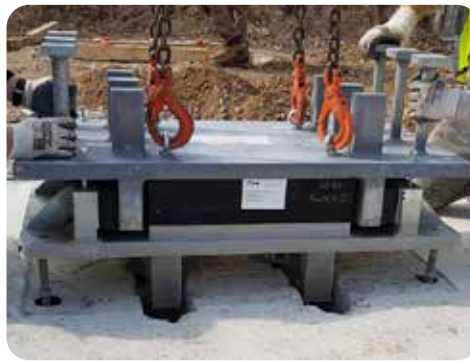
Fig 5.3 Farrat 700 kN Shear Key Unit Being Installed Into Pile Cap
