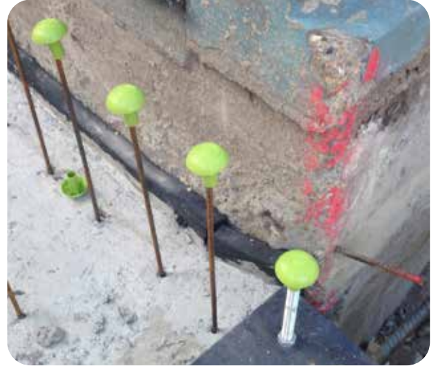
Fig 10.7 50 mm Thick Farrat ISOFOAM IS12
