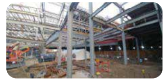
Fig 9.7 Steel Frame During Construction
