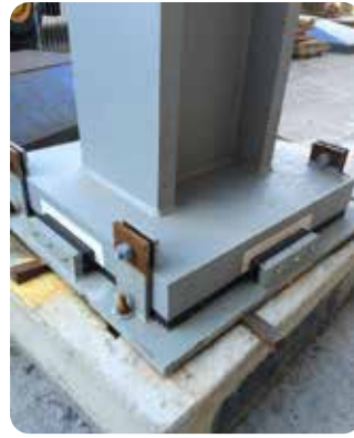
Fig 9.5 Isolation Bearing Assembly With Temporary Construction Restraints
