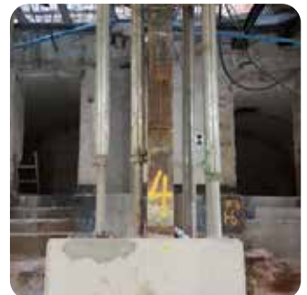
Fig 9.4 Isolation of Retained Façade
