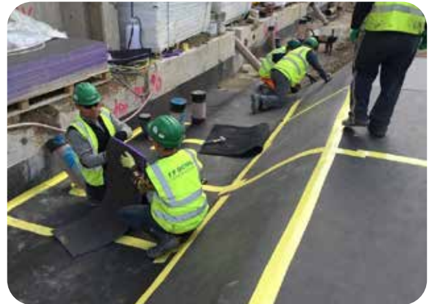
Fig 10.8 Verlimber Isolation Mat During Installation
