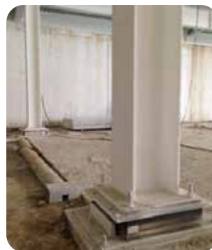
Fig 3.3 & Fig 3.4 Farrat LNR Bearings Supporting Steel Frames
