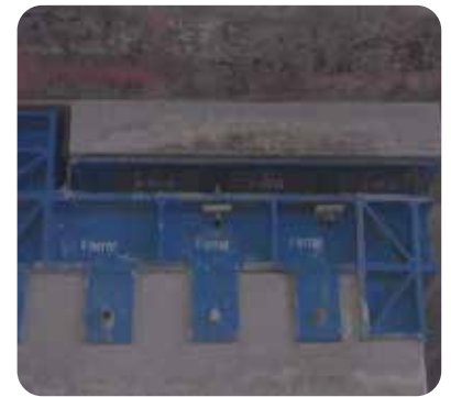
Fig 5.4 Farrat 2,000 kN Column Head Shear Key For Offset / Walking Column
