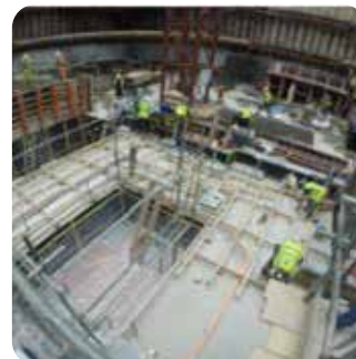
Fig 9.3 Construction of Cores
