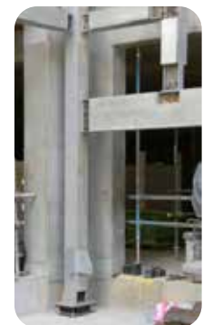
Fig 3.3 & Fig 3.4 Farrat LNR Bearings Supporting Steel Frames
