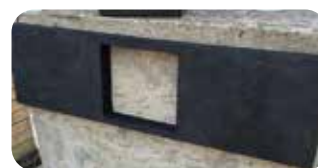
Fig 5.11 Self-Adhesive ISOFOAM with Pocket Cut Out to Accommodate Lateral Restraint Bearing
