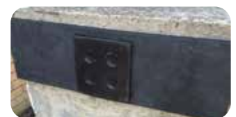
Fig 5.12 Lateral Restraint Bearing Within ISOFOAM Pocket
