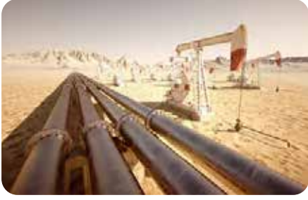
Sahil & Shah, Abu Dhabi Equipment Type: Compressors *Case study on Page 24
