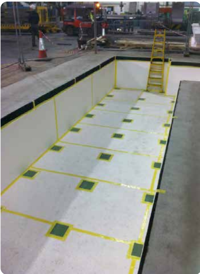
Fig 7.20 ISOMAT IFD with ISOFOAM Top Strip
