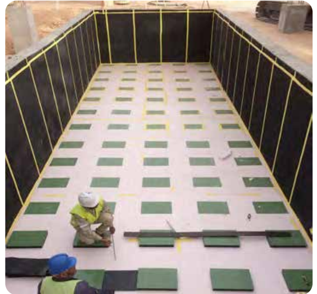
Fig 7.2 Example IFD Pit Using ISOMAT
