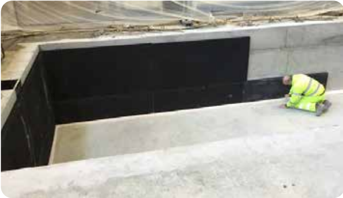
Fig 7.19 Farrat ISOFOAM Side Wall Isolation
