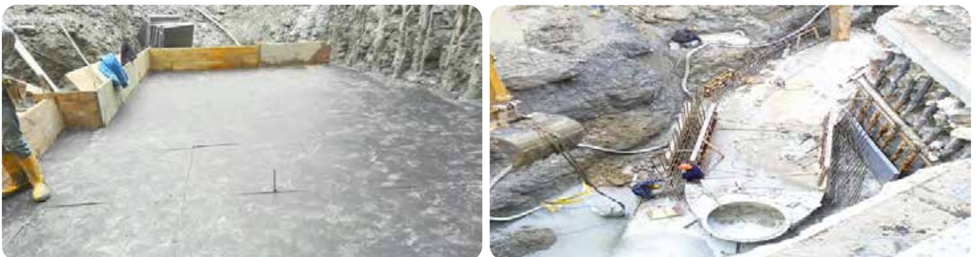
Fig 7.9 IFD Full Area Isolation Matting for a Water Turbine
