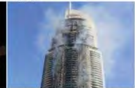
(f) The Address building (Dubai) after the fire
