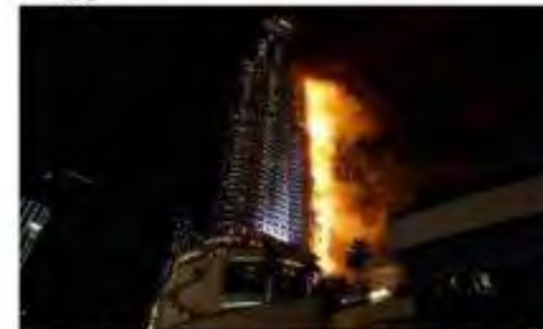
(e) The Address Building (Dubai) during the fire
